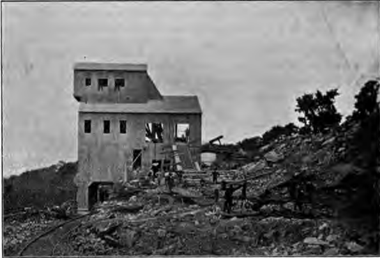
Limestone Crusher From a photograph
